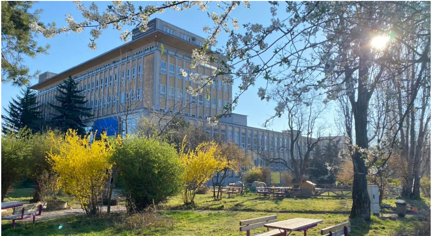
Photo: A view of the Nová Cvernovka building
